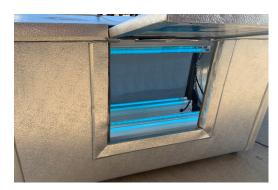
The science of the AIRrowSwift incorporates UV-C technology into existing air conditioning and filtration systems for small buildings, warehouses, as well as tents, trailers, and other facilities. The UV-C technology eradicates particles and viruses in the air as it passes through the AIRrowSwift chamber prior to allowing them to circulate through air vents.
